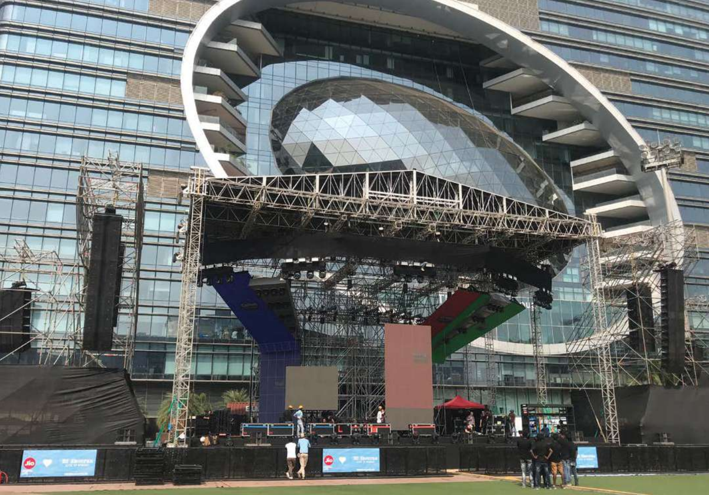
A unique cantilever over a cantilever was built for the Ed Sheeran show, with 15 cantilevers being built on a single structure and another 4 over them. This was also the first time a Layher based cantilever was built for the main PA too
